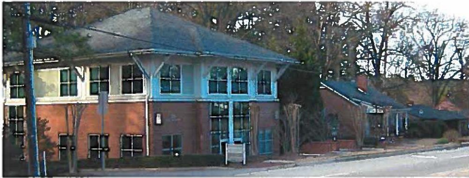
Figure 6-5-8: Similar building materials to adjacent single-family dwellings
