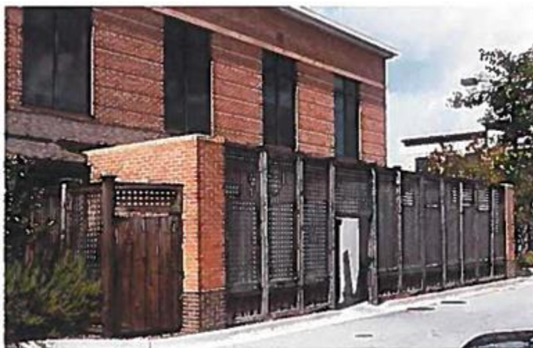
Figure 6-5-9: Screening elements integrated with the building
